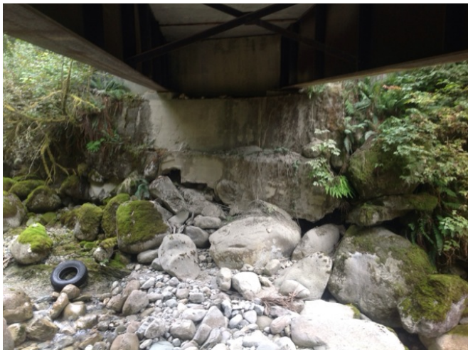
Left Bank Abutment when facing downstream
