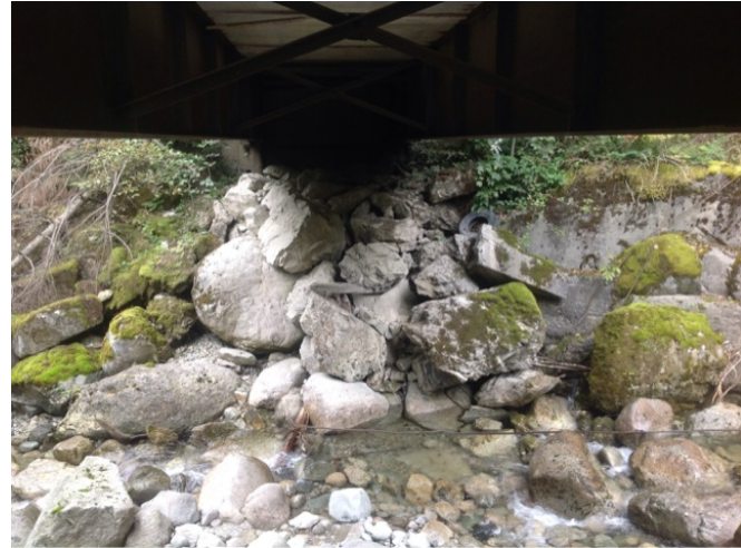
Right Bank Abutment when facing downstream
